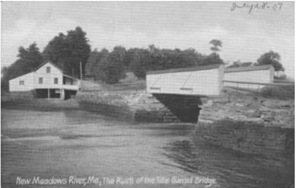
Gurnet Bridge July 28, 1907
