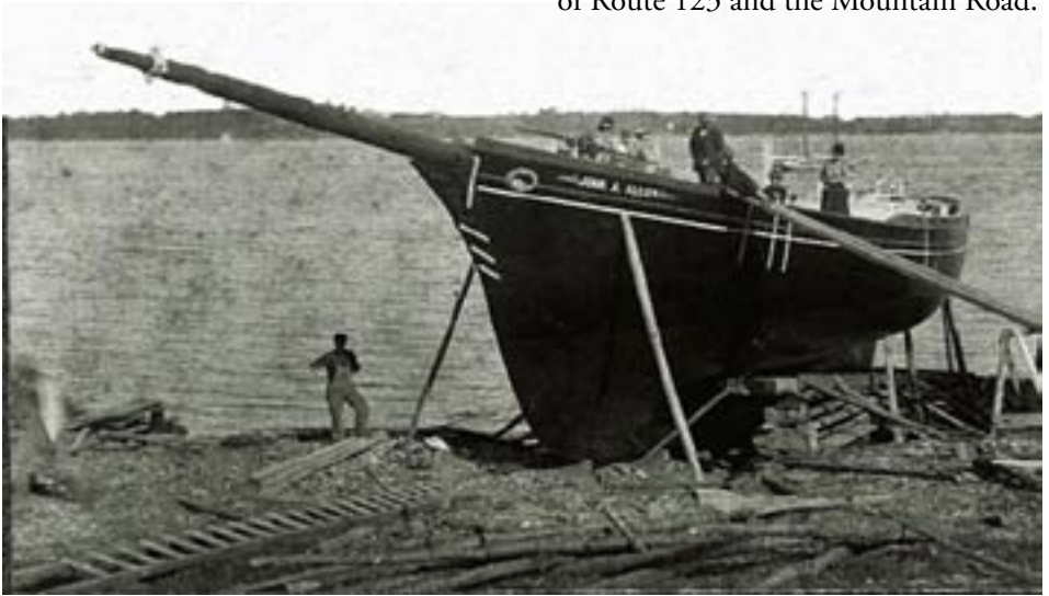
Schooner John A. Allen nearly ready for launch from the Allen shipyard, Clark's Cove, Harpswell, Maine, 1902. The ship carpenter standing on the shore was Freelon Smith—the other individuals standing on the deck are unknown, but probably included some of the Allen family.
