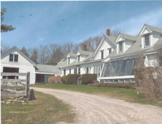
Former Holbrook house on Peabody Rd
